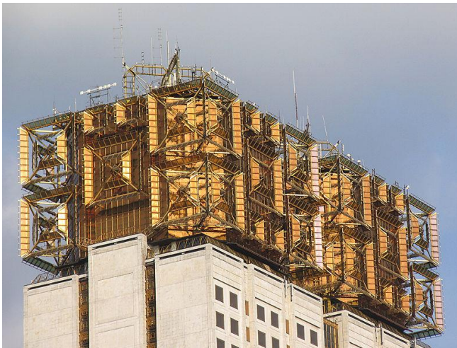
Fig. 4. Solar batteries on the roof of Science Academy of Russia
