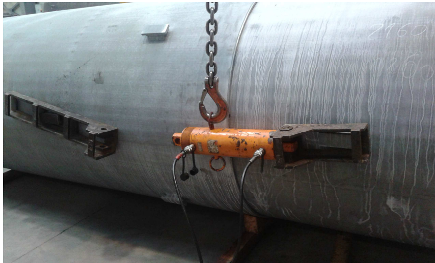
Fig. 1. Assembly of the steel shell tower trunk
