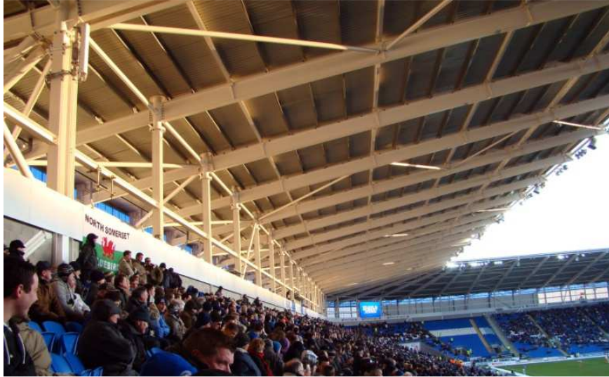
Fig. 2. Stand roof structure of Cardiff City Stadium, Cardiff, Wales (author of photography: Jon Candy [10])
