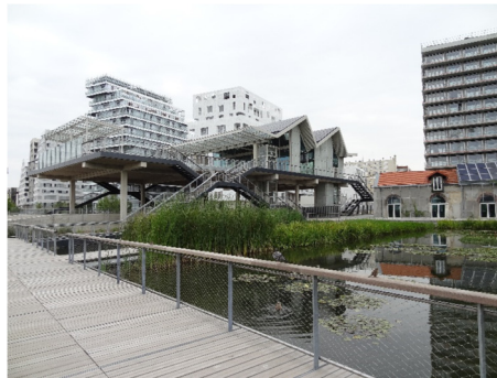
Fig. 9. Martin Luther King Park in Paris. Elevated platform with shelter build over highway crossing. Photo: Monika Trojanowska
