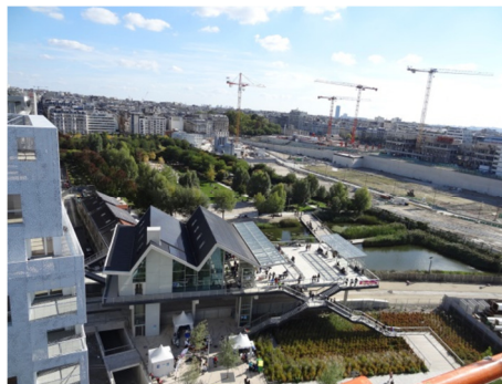
Fig. 5. Martin Luther King Park in Paris. Pavilion and platform built over highway crossing. Photo: Monika Trojanowska
